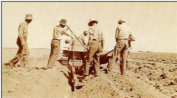
Irrigation Ditch Construction
